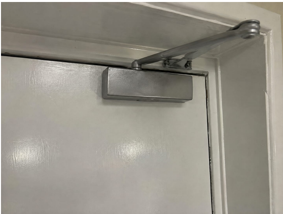
Overhead self-closer, communal entrance door
