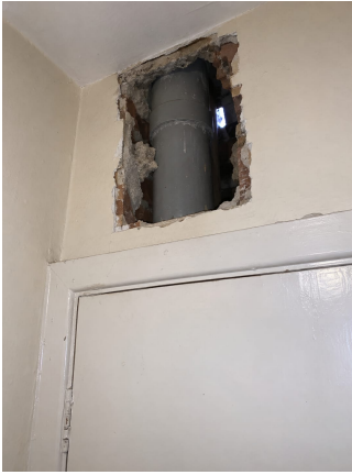
2nd floor lobby
