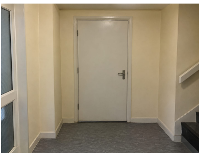
Ground-floor flat entrance door
