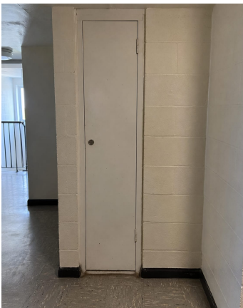
First-floor riser cupboard door
