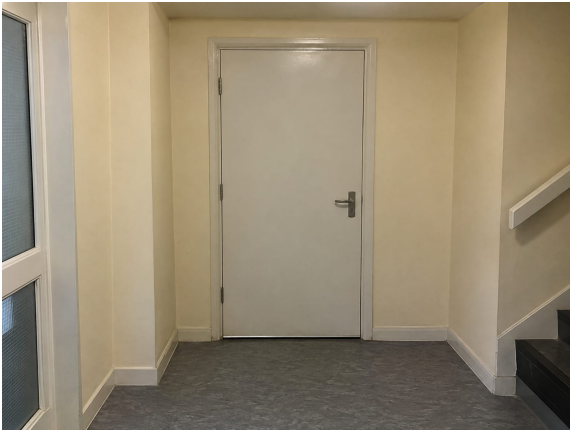
Ground-floor flat entrance door
